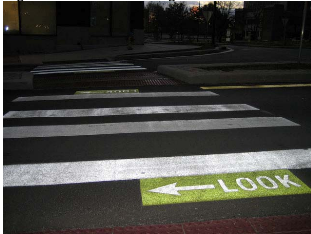
Figure A5. Pavement Legends for Pedestrians
